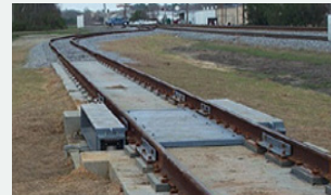
This certified Coupled-in-Motion Scale is made by Systems Associates, Inc.
